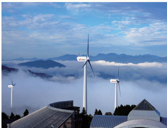
Shikoku Electric Power's wind power generation facility installed at Yutoristo Park Otoy, an outdoor recreation and tourism facility in Otoy Town, Kochi
