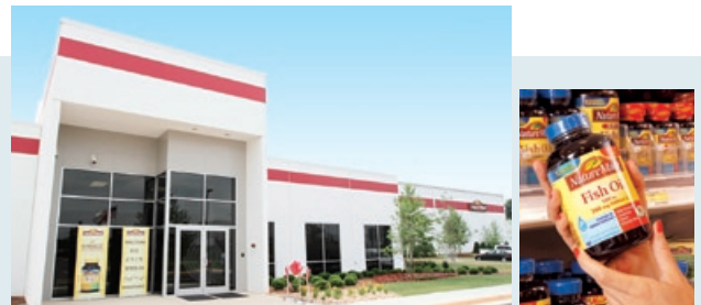
Pharmavite LLC (Northridge, California)
