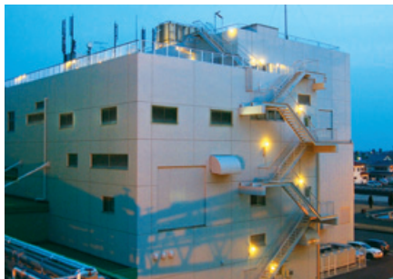
Otsuka Pharmaceutical Factory: Emergency LED lights along evacuation routes and at evacuation sites automatically turn on during a power outage.
